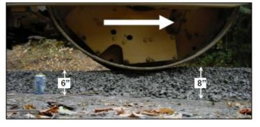
4. Vibratory Roller: The first roller pass over all aggregate should be done in static mode (vibration turned off) to "set" the aggregate, and Figure 16. A roller moving from left to right compacts the successive passes should be done in
