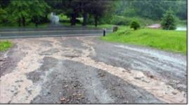
Figure 19. Water in wheel tracks.
