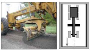
Figure 30. Grader leaving the road with a high flat center.
