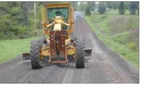
Figure 29. Material is knocked down
