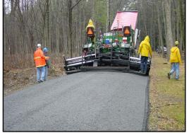
**Figure 15.** Paver placement of DSA with proper crown.
