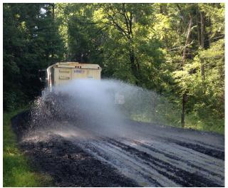
Figure 27. Adding water to a dry road surface.
