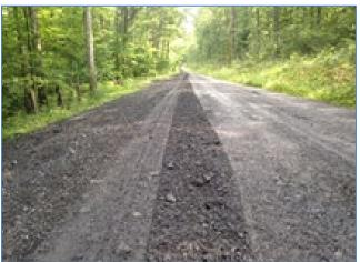
Figure 32. Before & after first pass of 10-ton roller.
